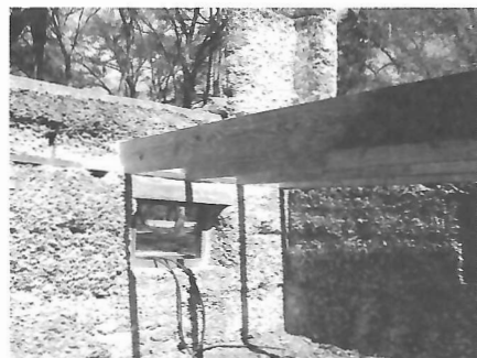
West wing floor joists
