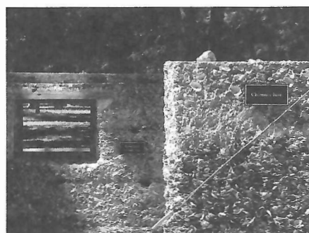
Chimney base in lower-level storage area.
